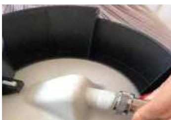
**3 |** Screw the hand shower onto the supplied hose with the appropriate gasket.
